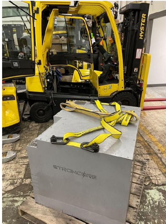
Figure 16: Image of 4x M14 lifting hoists and three (3) lifting straps secured on the battery.
