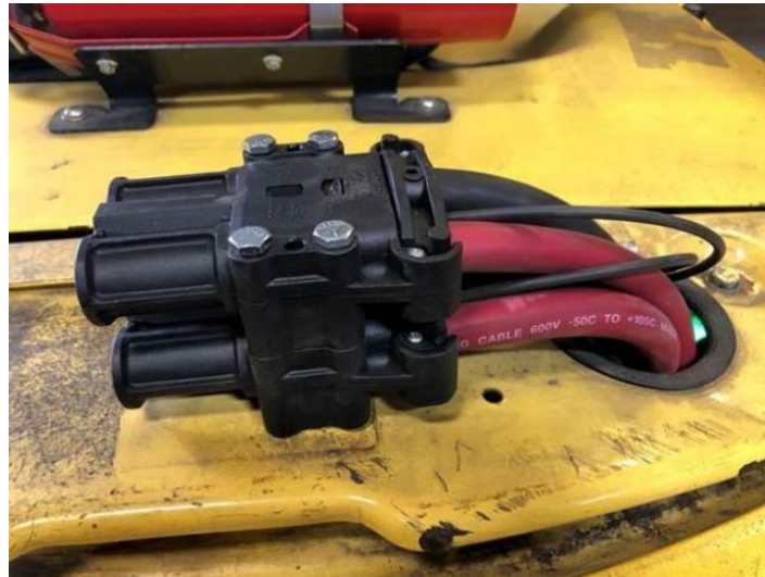
Figure 21: Image of charge jumper cable routed to back of forklift and connectors secured on chassis of the forklift.
